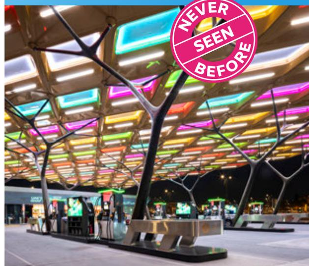
The UAE's national tree is renowned for its resilience to harsh weather conditions. The Service Station of the Future is built on an exoskeleton based on the ghaf tree structure, supporting a cutting-edge, solar-powered, carbon-fibre canopy.
